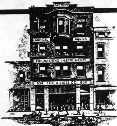
The A. Lietz Company at 632 Commercial Street in San Francisco before the earthquake and fire of April 18, 1906.
