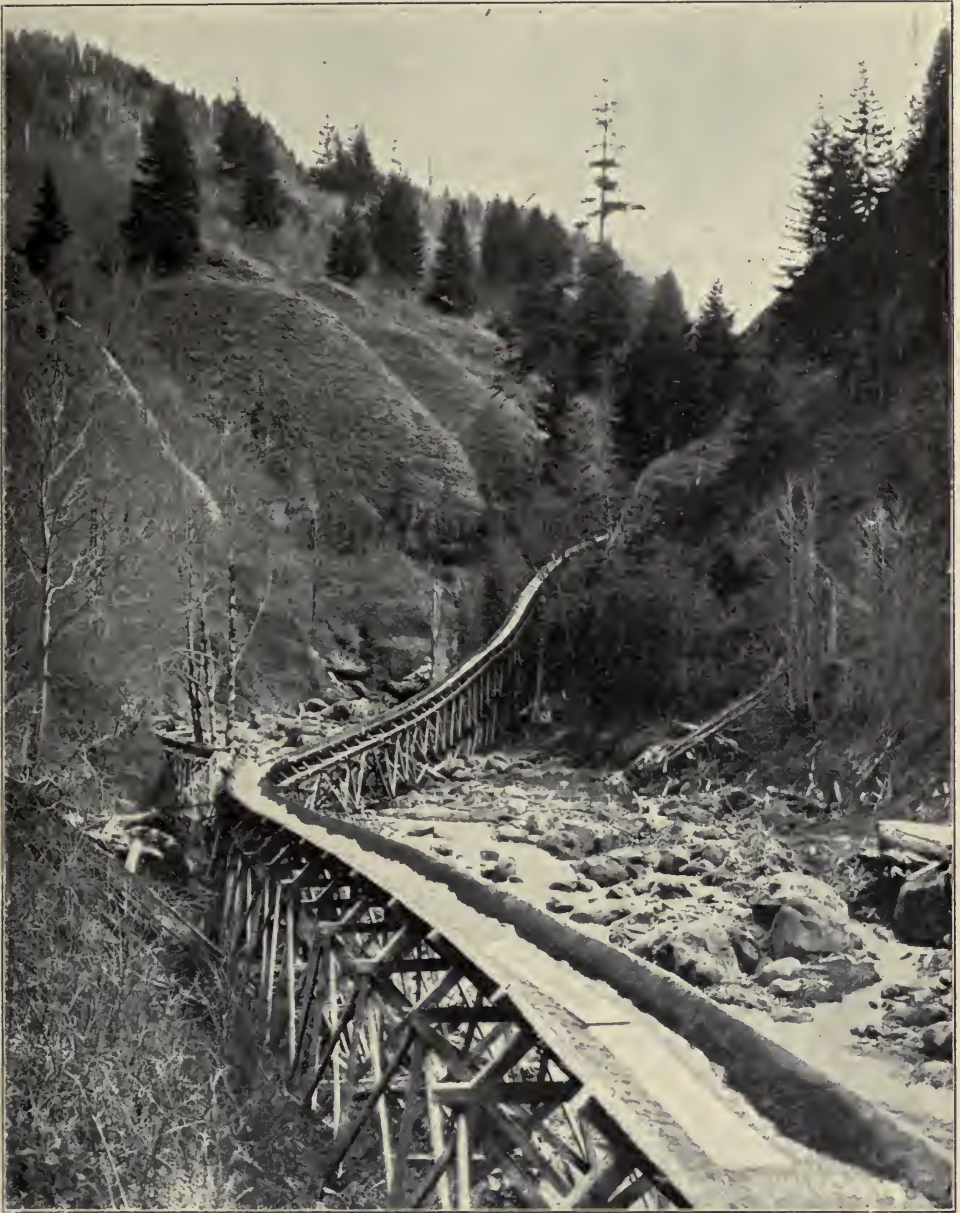
Lumber flume at Bridal Veil, Oregon, having a drop of 2,500 feet in two miles. Timbers 12x12 and 60 feet in length have come down this flume
