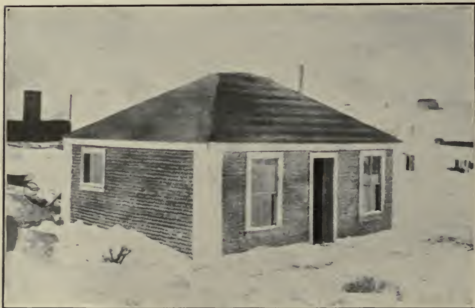
House made of beer bottles in Tonopah Nevada. Ten thousand bottles incorporated in structure
