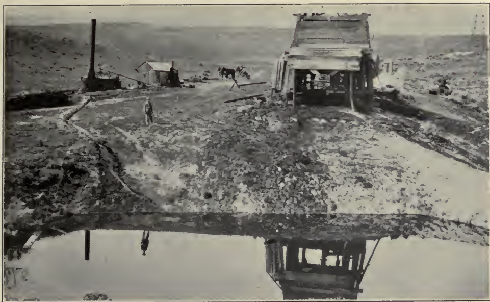
Standard drilling rig in operation, showing a "sump hole" where the oil is stored after a gusher has been struck
