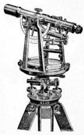
The dimensions are as follows: Horizontal limb, 5 inch, with graduations on Solid Silver, with two double Verniers reading to single minutes; 5 inch Vertical Arc with Clamp and Tangent, Level under Telescope; Magnetic Needle, 3 % inches long; Telescope, 9 inches, with a power of 20 diameters and an exceedingly flat field; Extension Tripod with Thumb Nuts; weight of Instrument, complete with Tripod about 16 pounds.
