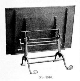
This is a rigid table of graceful design, and is easy of adjustment, having a tilting movement from horizontal to perpendicular, and can be adjusted in height from 30 to 45 inches, the greatest height of any table made.
