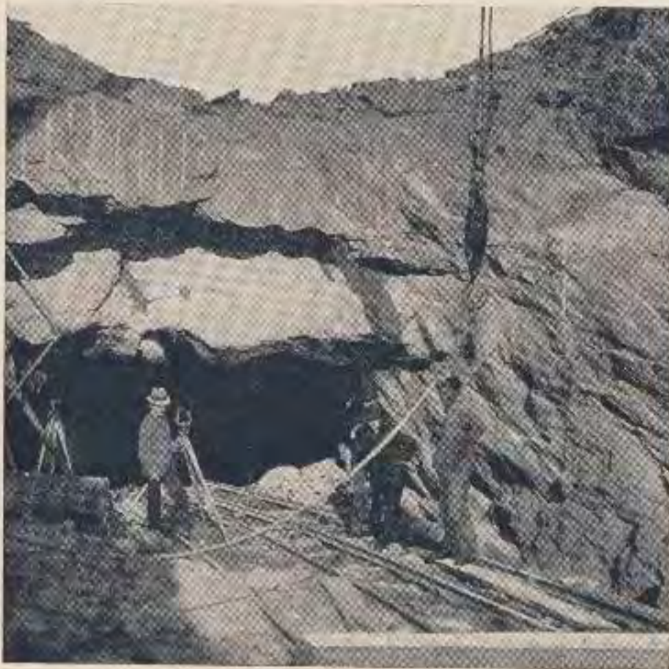
RAPID TRANSIT TUNNEL EXCAVATION, NEW YORK CITY.
