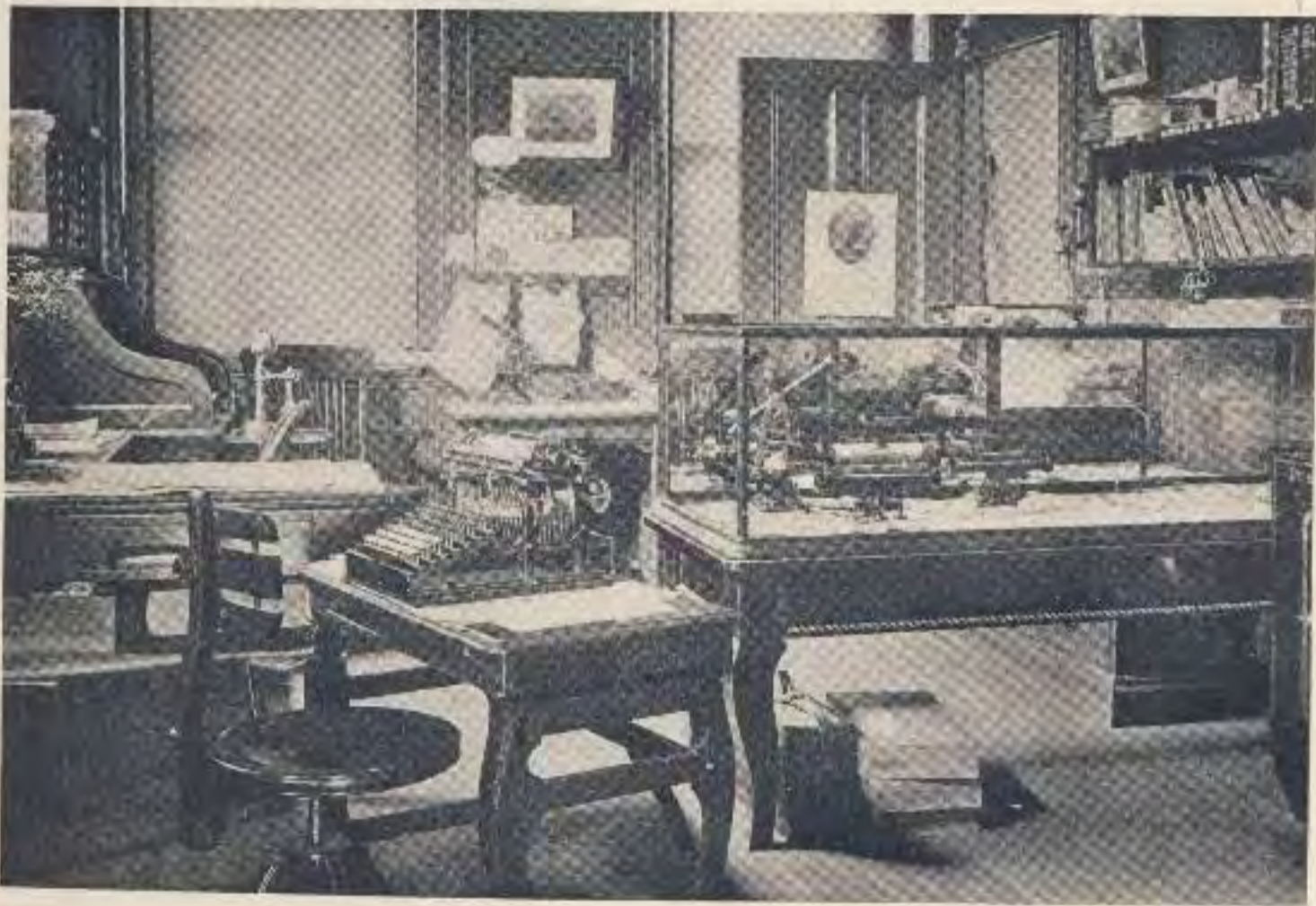
NORTH END OF GENERAL OFFICE.
