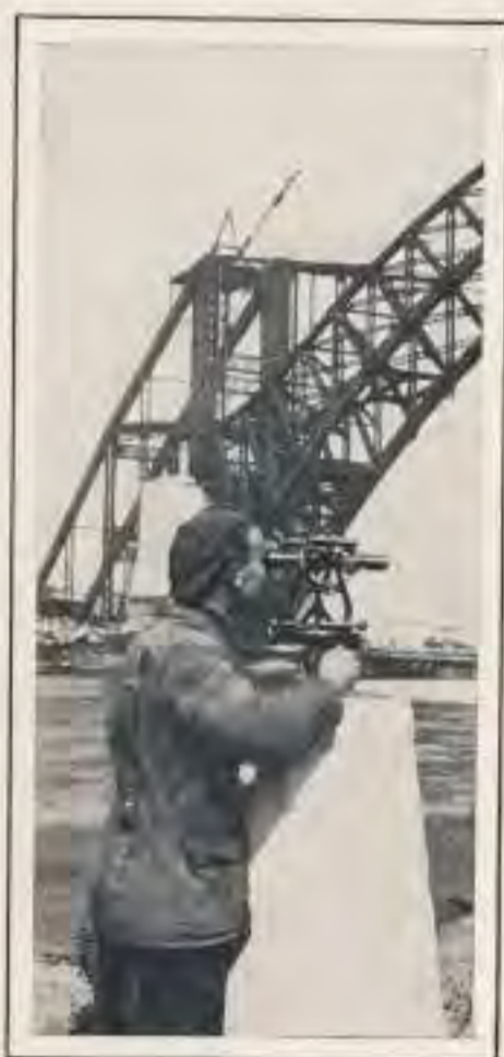
Gutley Precise Transit No. 18-A, mounted on concrete pier, as used at Hell Gate Bridge See pages 28 and 29.
