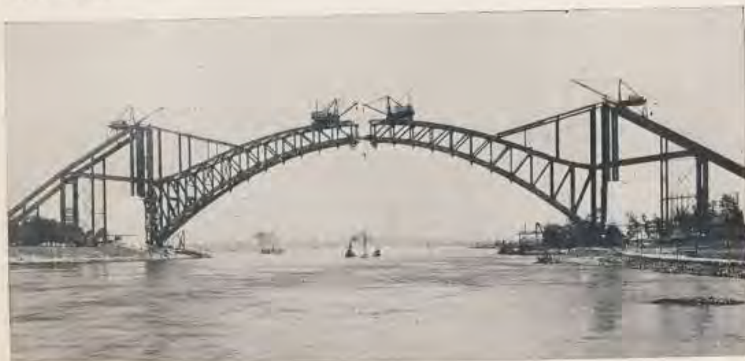
View of Hell Gate Bridge during construction
