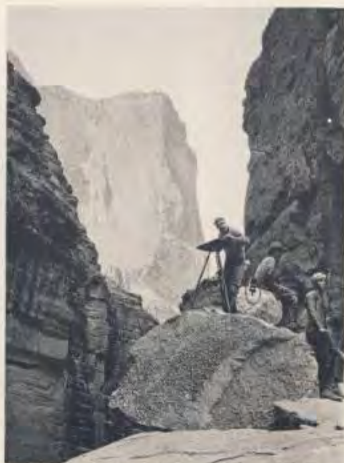
A U. S. Geological Survey Party using a Gurley Plane Table Outfit in mapping the Grand Canyon of the Colorado.
