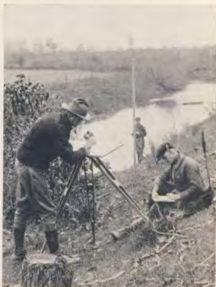
Plane table method produces accurate, rapidly-made maps showing all topographic features.
