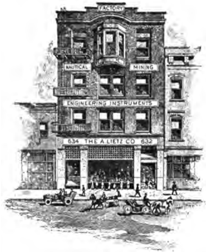
THE A. LIETZ CO. BUILDING Before the San Francisco Catastrophe of April 18, 1906.
