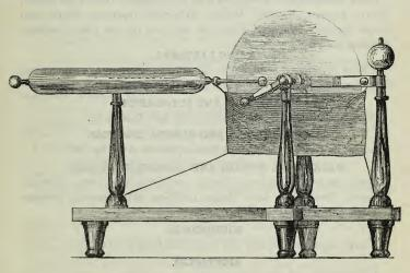
Plate Electrical Machines 16 to 36 inch plates, \$20 to \$125; Leyden Jars, Batteries, Dischargers, Dancing Plates, Chime of two three and five Bells, Electrometers, Insulated Stools, Aurora Tubes, Electrical Pistols, Cannons, Orreries, Heads of Hair &c., Thunder Houses, Luminous Words, Misers' Plates, Egg Stands, Tin Foil, Amalgam, Brass Chain, &c. &c.
