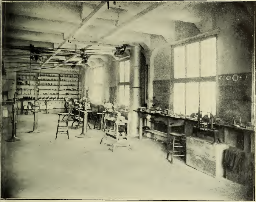
ASSEMBLING AND ADJUSTING DEPARTMENTS, Third Floor.
