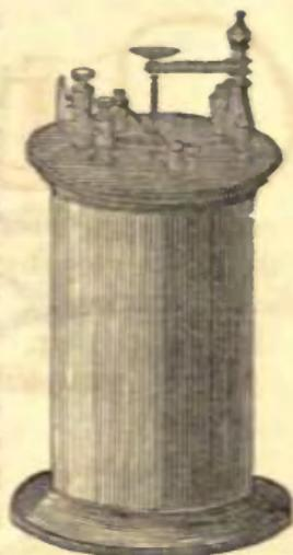
*Saxton's Magneto-Electric Machine.*—(Fig. 478, next page.)—The magneto-electric machine is one of the most interesting and instructive instruments of modern science; by it we see exemplified the close connexion between, if not the identity of, the electric and magnetic forces; by it the same heating, magnetizing, and decomposing power, the same chemical effects, are shown to be common to both.
