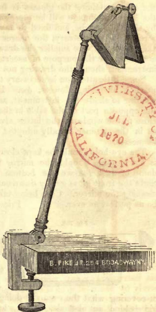
If objects can be seen distinctly on the upper part of the paper, and not on the lower, incline the part of the case reflected downwards by the joints, until the reflected image is on the part of the paper required. Many persons, upon first attempting to use the instrument, occasionally lose sight of their object or pencil by an unintentional motion of the eye; to avoid which, contract the eye-hole by means of the eye-piece which covers it.
