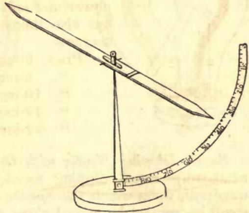
*The Astatic Needle.*—(Fig. 414.)—Two needles, perfectly similar in their form, and magnetic intensity, are turned with their poles in opposite directions, and placed upon the same axis perpendicular to their length.
