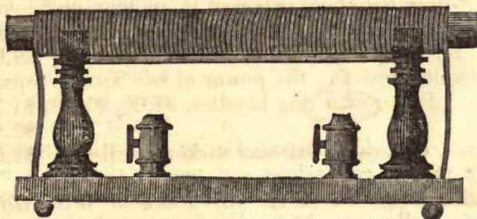
*Helix on Stand.*—(Fig. 428, as above.)—The helix consists of a coil of insulated copper wire, bound in the form of a close spiral spring, in one or several layers, so as to form a hollow cylinder, into which an iron rod or any body to be magnetized, is to be placed. Those having a number of layers, and the internal diameter small, have great magnetizing power.
